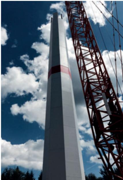
Patented Ventur hybrid tower for wind turbines
