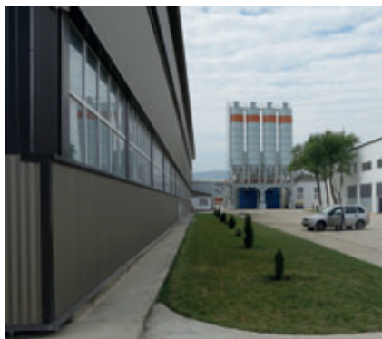
View of the building façade with the adjacent concrete mixing plant
