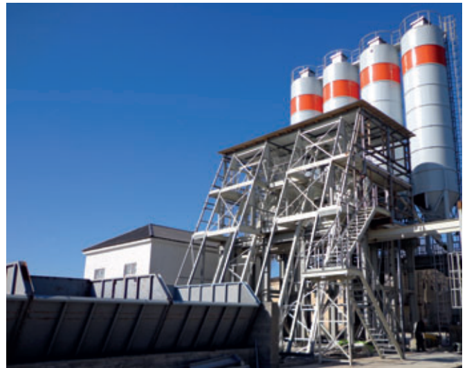
Teka mixing plant during the construction phase
