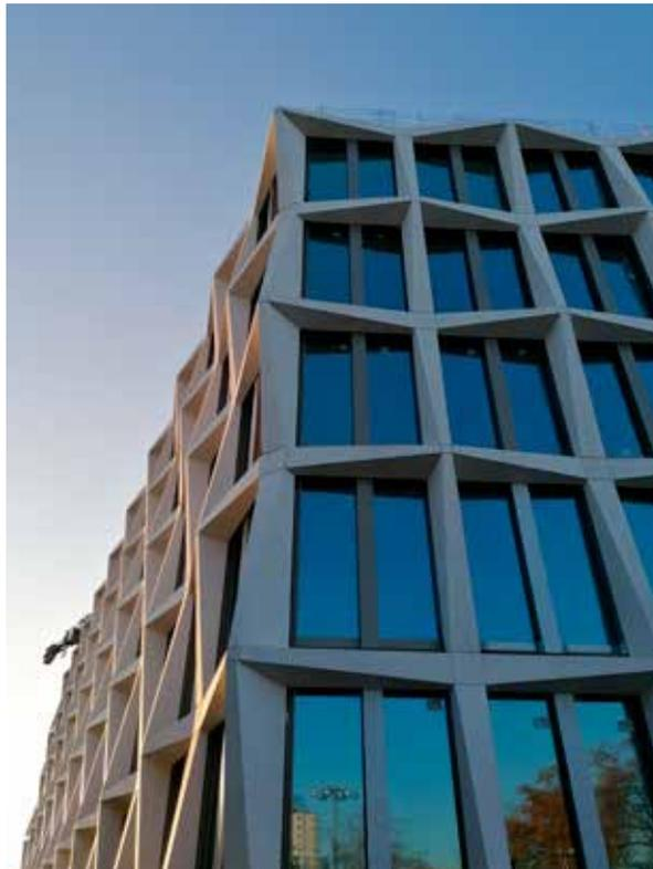
BWE-Bau delivered the load-bearing precast external support structure for the Neuer Kanzlerplatz project in Bonn
